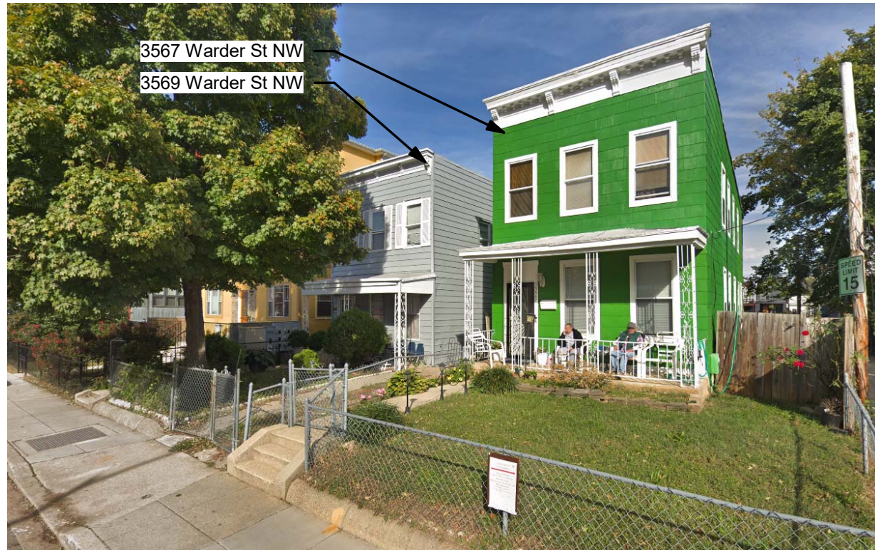
FROM STREET (SHOWING 3567 WARDER ST NW)
