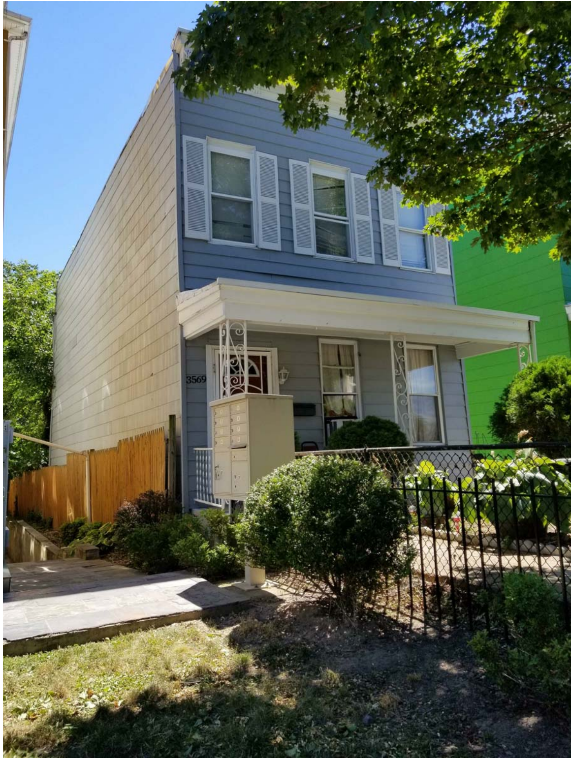
EXISTING FRONT PORCH CONDITION
